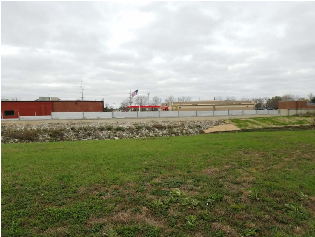
Figure 2: Floodwall east of Pump Station 10 as viewed from the north side of Clear Creek
