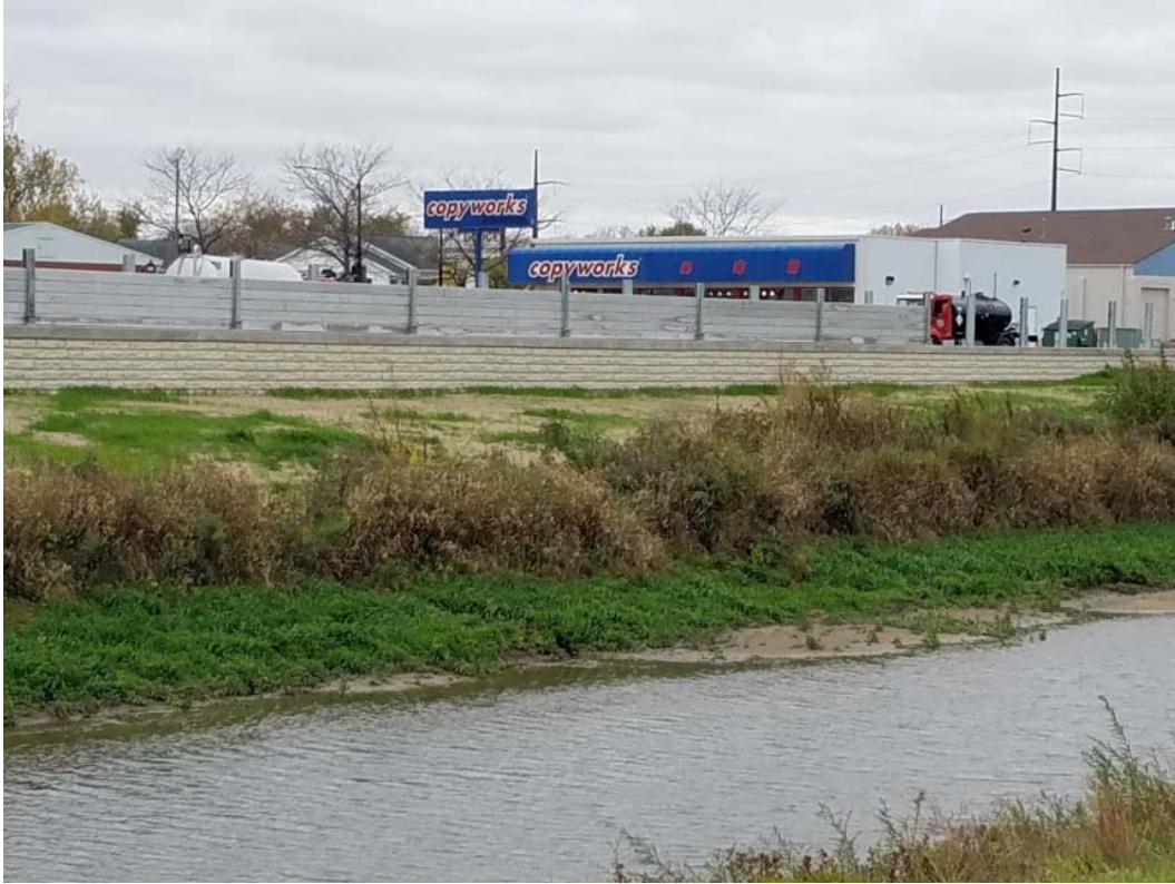
Figure 1: Floodwall west of Pump Station 10 as viewed from the north side of Clear Creek
