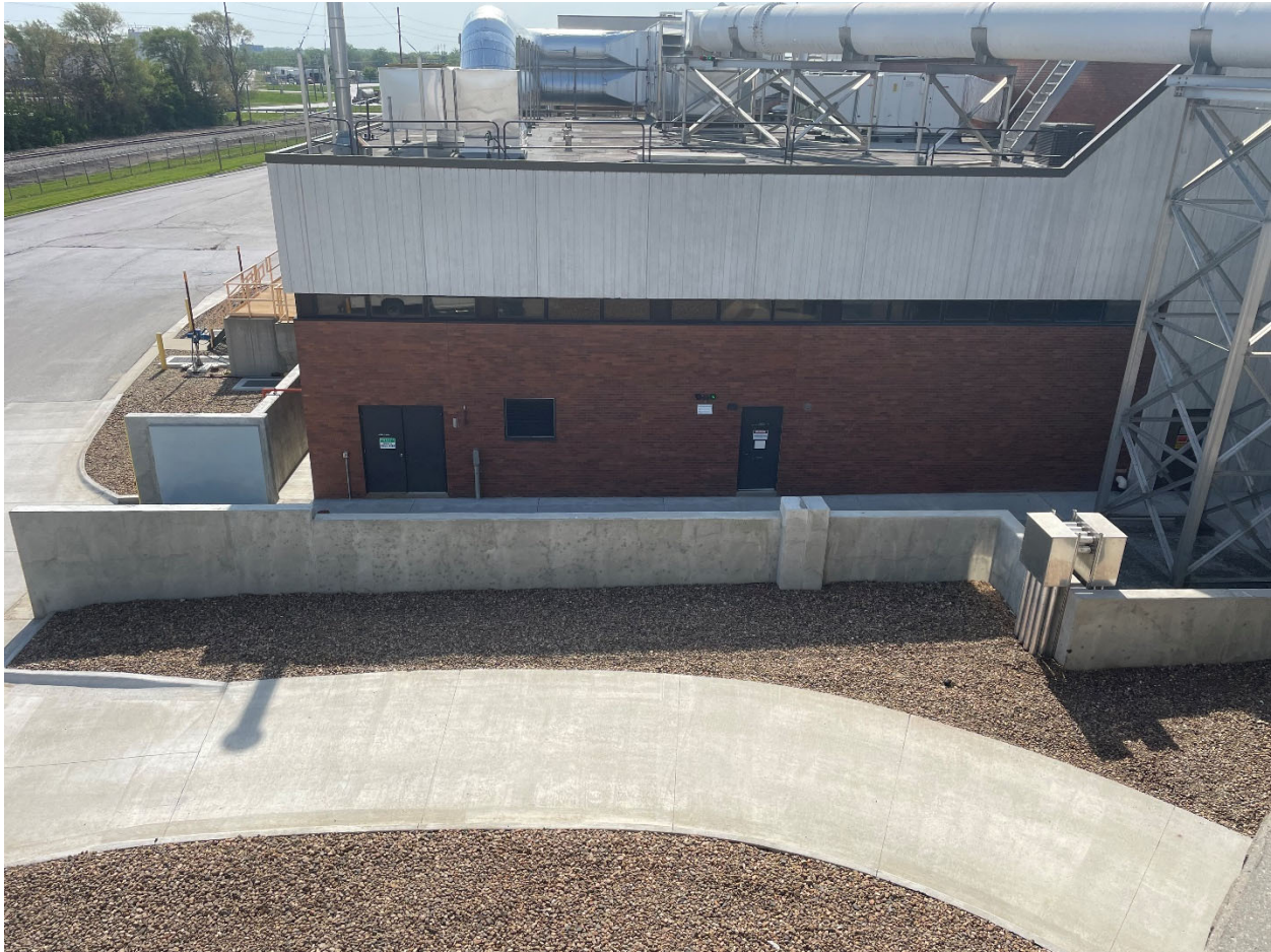
Figure 4: Flood Wall on West Side of Main Pump Building
