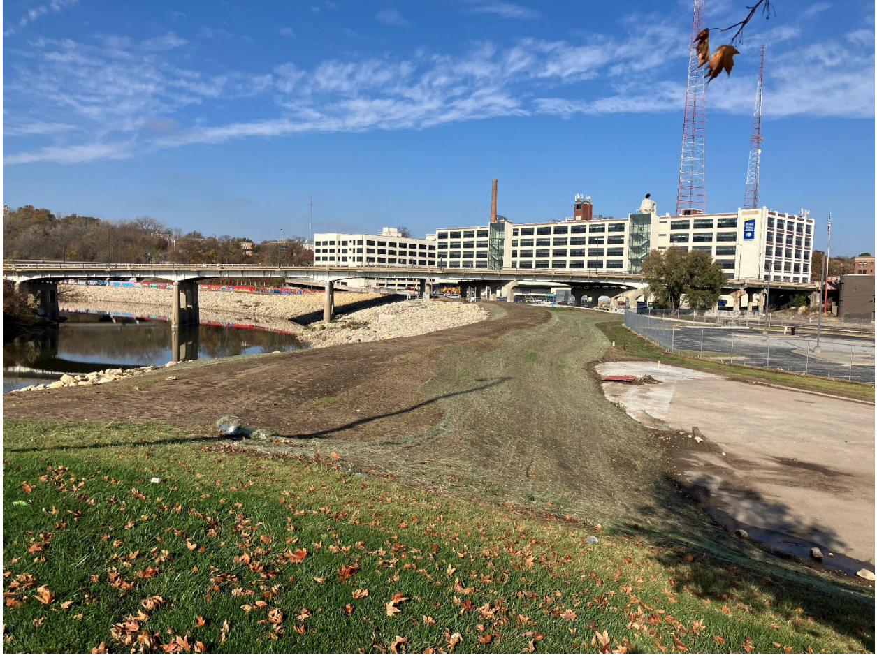
DSM Levee Alt Phase B north of MLK Bridge
