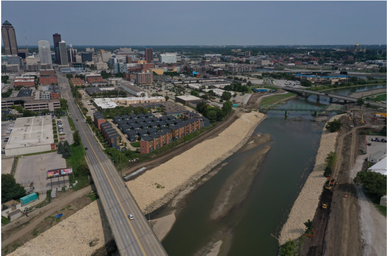
Photo from Parks and Recreation drone above SW 7 th Street bridge looking down stream
