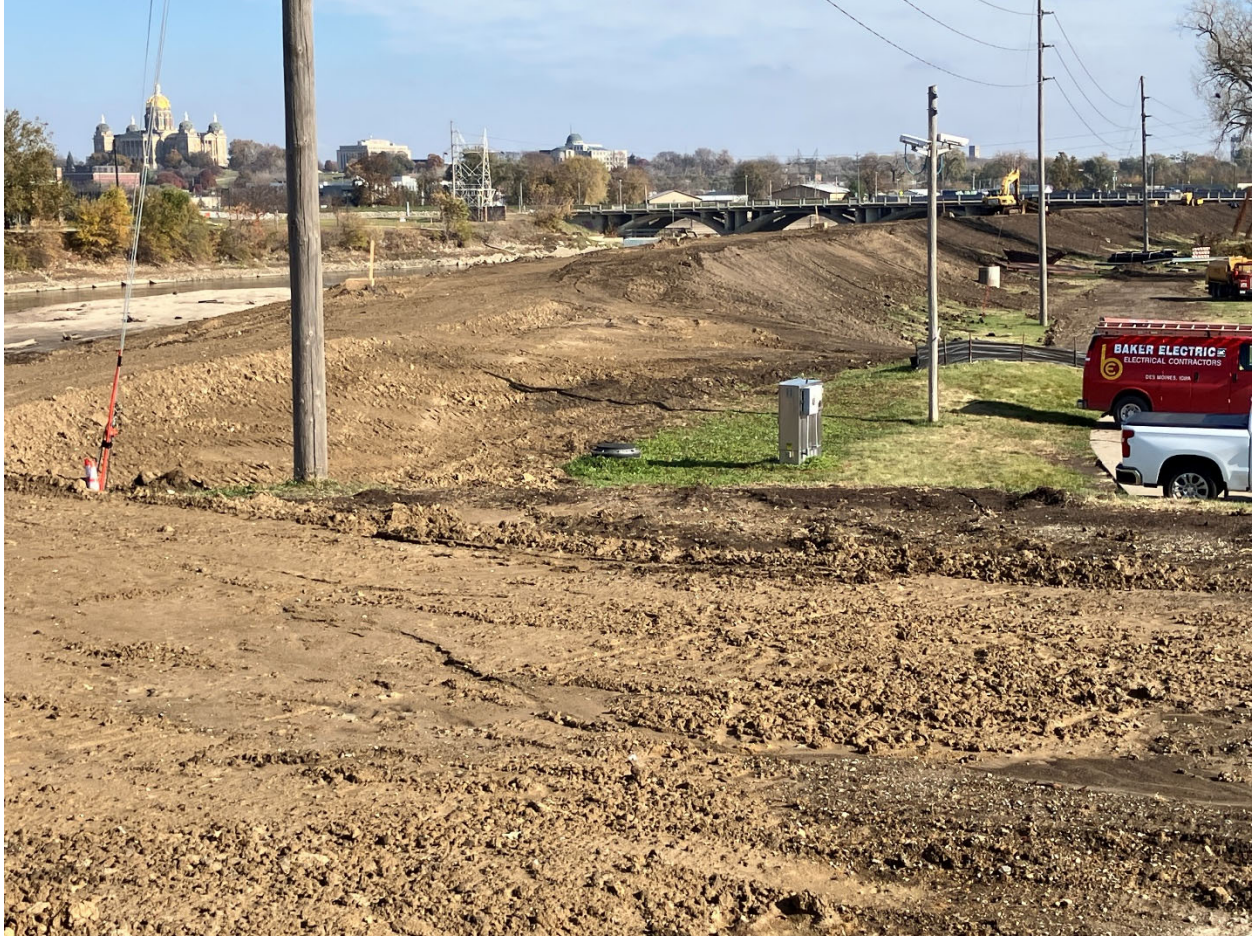
DSM Levee Alt Phase C, south side
