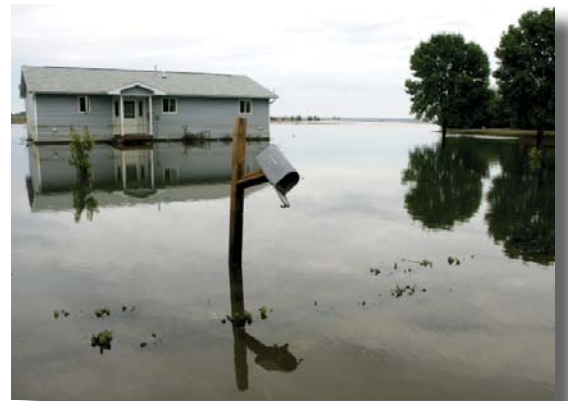
Oakville home surrounded by flood waters in 2008. FEMA photo.
