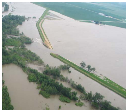
Levee near Hamburg in Fremont County, June 13, 2011.
