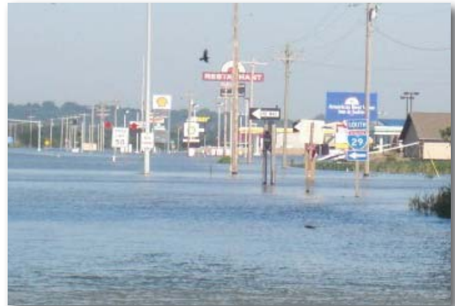
Flooding of the Missouri River at Highway 2 and I-29 in Fremont County. Photo by Major Tim Leinen
