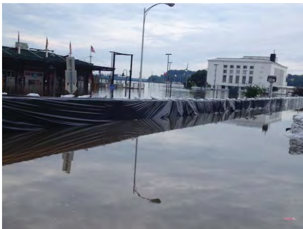
July 2014 flooding in Burlington.
