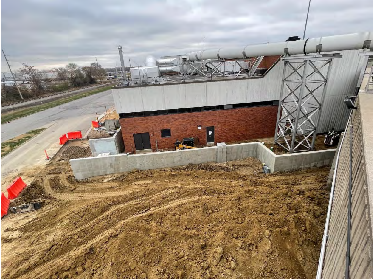
Figure 4: Flood Wall Under Construction on West Side of Main Pump Building
