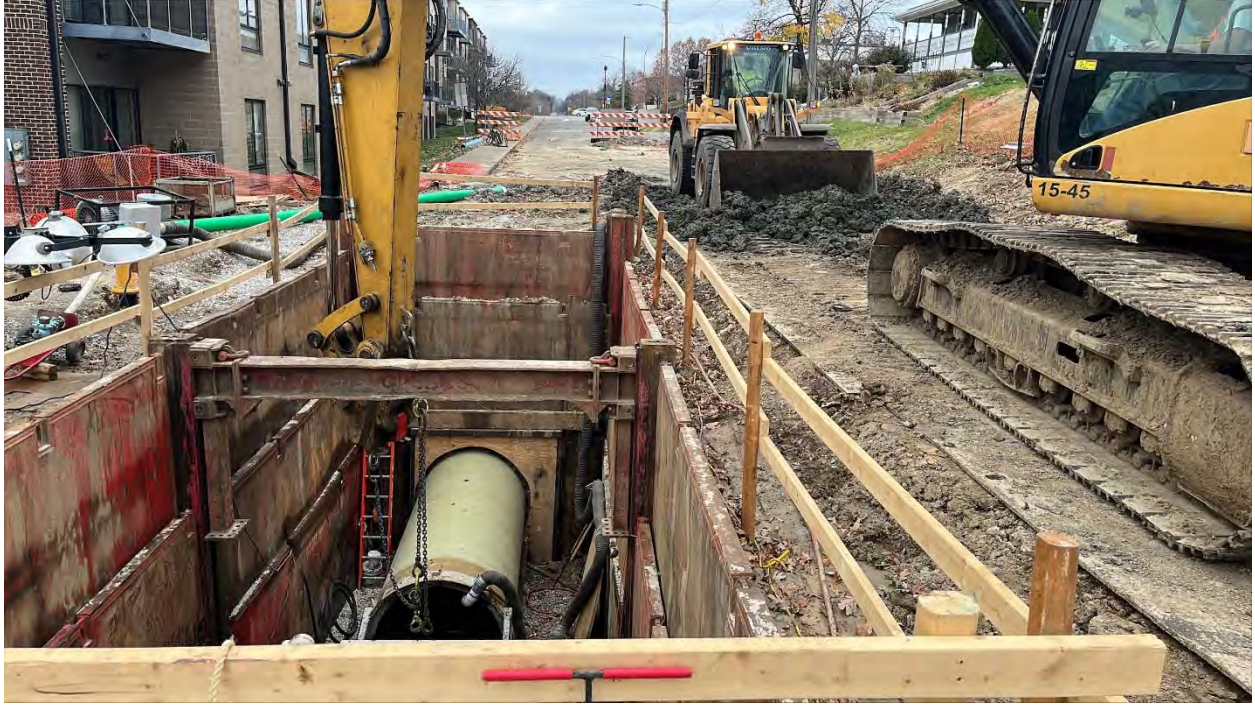
Figure 6: Segment 3 Pipe Boring Operation
