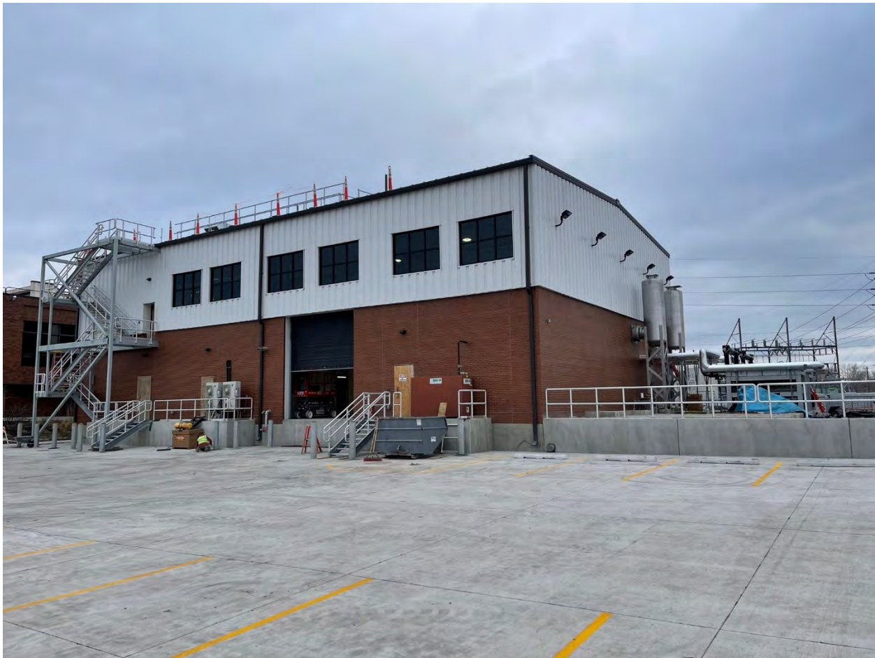
Figure 1: New Standby Power and Electrical Service Building
