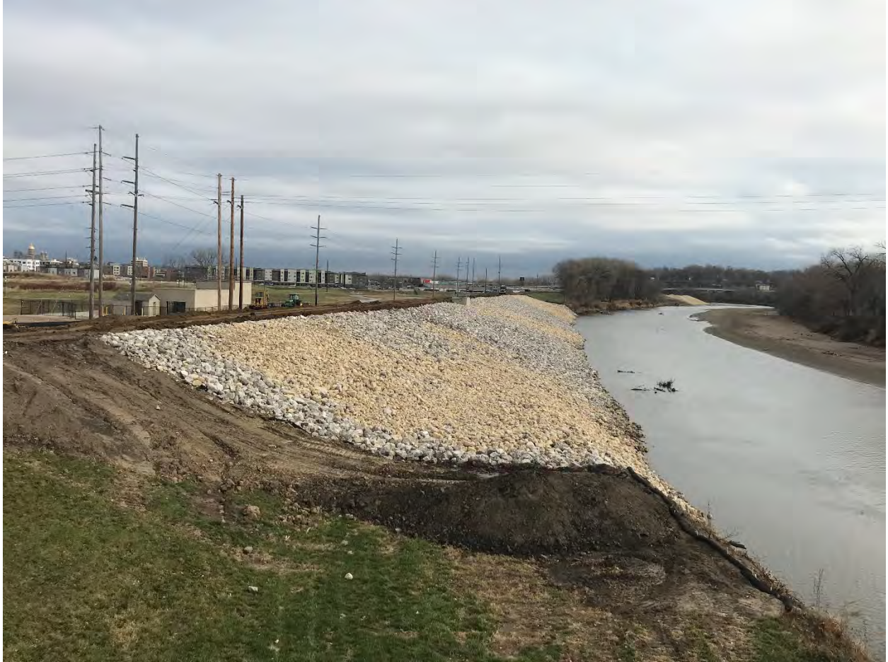
DSM Levee Alt Phase B, Phase 2, north side
