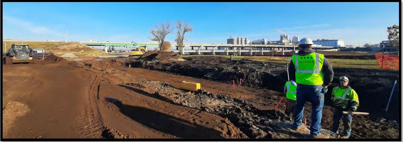
Figure 8. 1ST STREET SW FLOODWALL OCTOBER 2022
