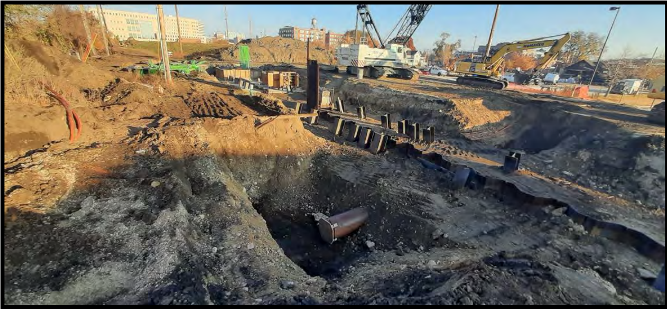
Figure 17. 12TH AVENUE SE SHEETING, H-PILE, AND WATERMAIN CASING PIPE OCTOBER 2022
