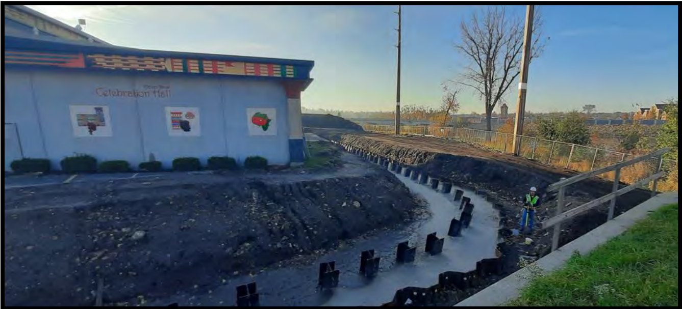
Figure 15. 12 TH AVENUE SE FLOODWALL PROGRESS OCTOBER 2022
