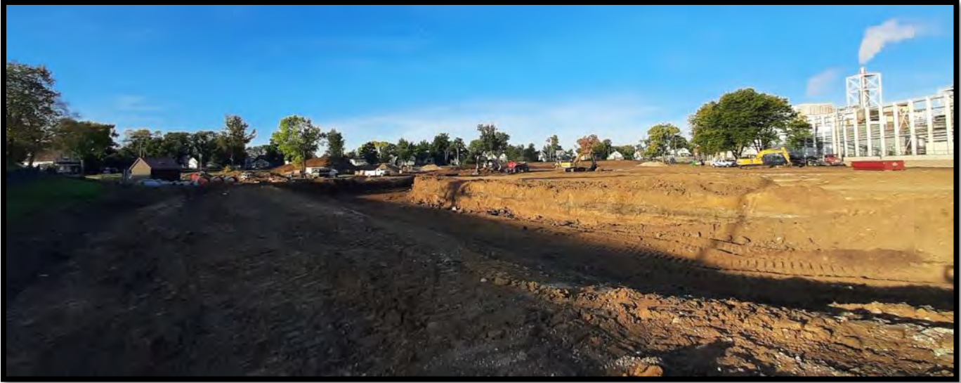
Figure 10. 12TH AVENUE SW DETENTION BASIN PROGRESS OCTOBER 2022
