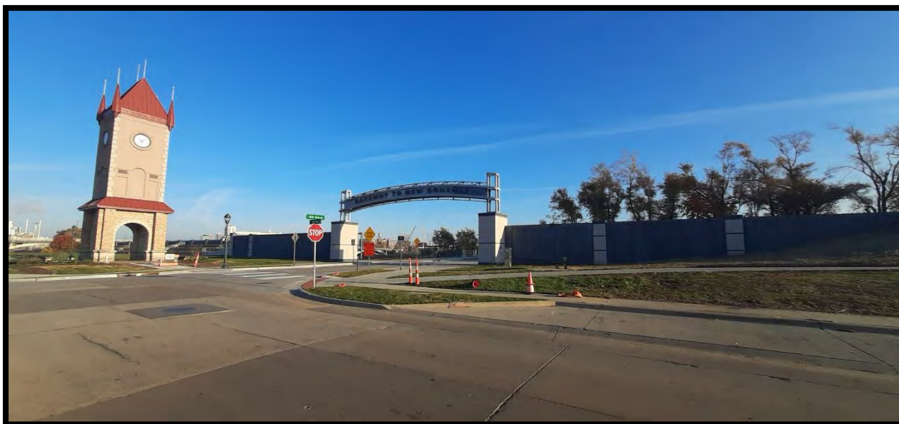
Figure 13. 16 TH AVENUE SW GATE AND FLOODWALLS
