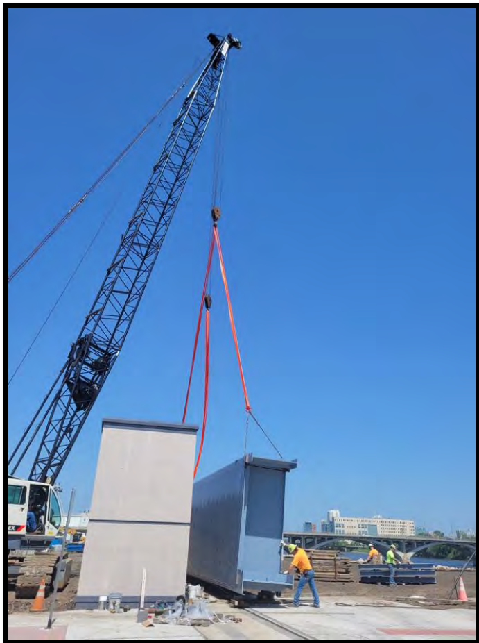
Figure 12. 16 TH AVENUE SW ROLLER GATE INSTALLATION
