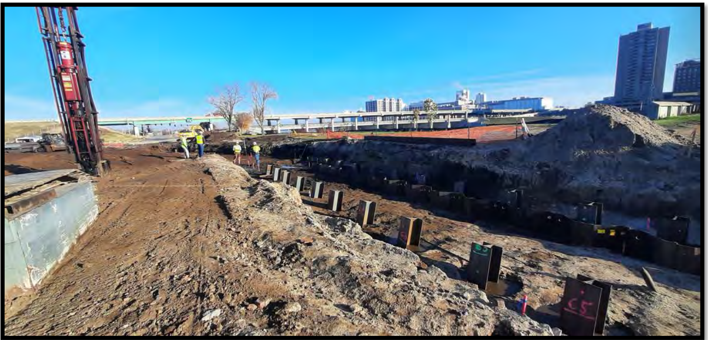
Figure 9. 1ST STREET SW FLOODWALL OCTOBER 2022
