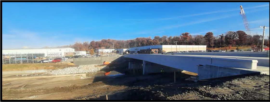
Figure 4. SHAVER ROAD NE BRIDGE AND FLOODWALL SEPTEMBER 2022
