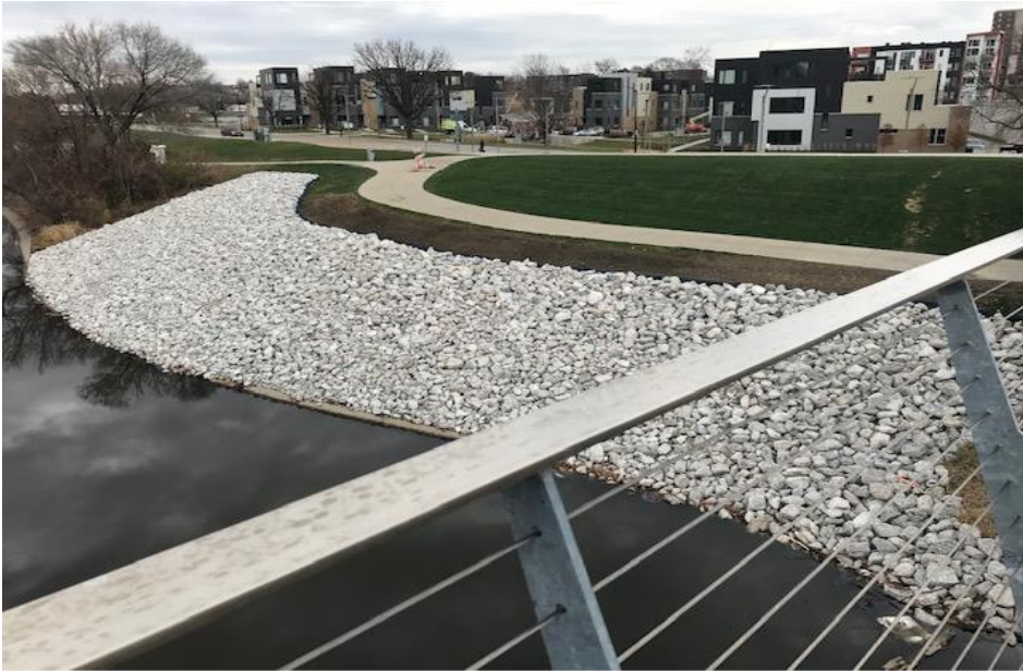
Northside of Women's Achievement Bridge
