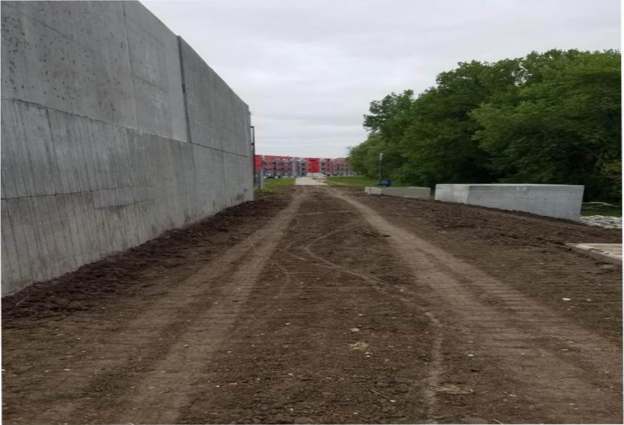
S.E. 4th and Van Buren Storm Water Pump Station Improvements
