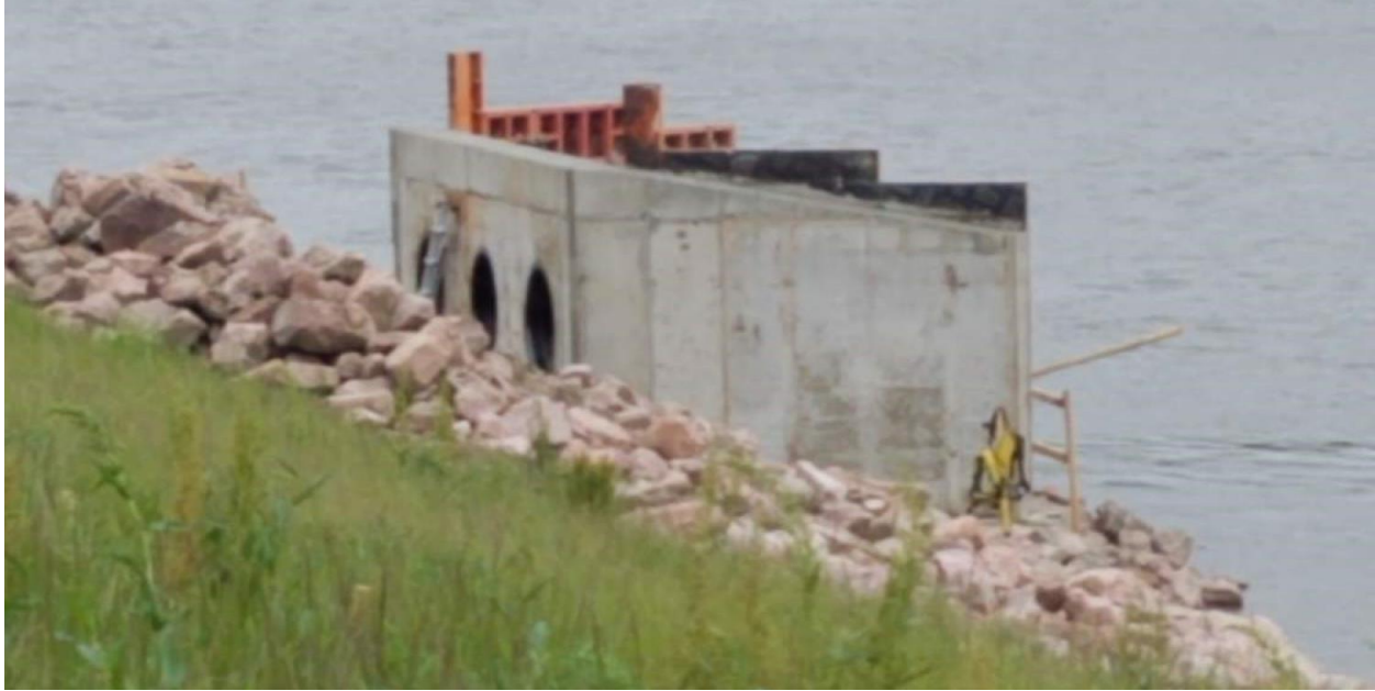
S.E. 9th Street Storm Water Pump Station and Improvements
