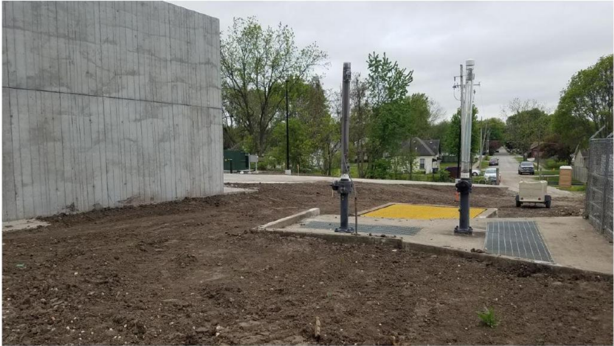
S.E. 4th and Van Buren Storm Water Pump Station Improvements
