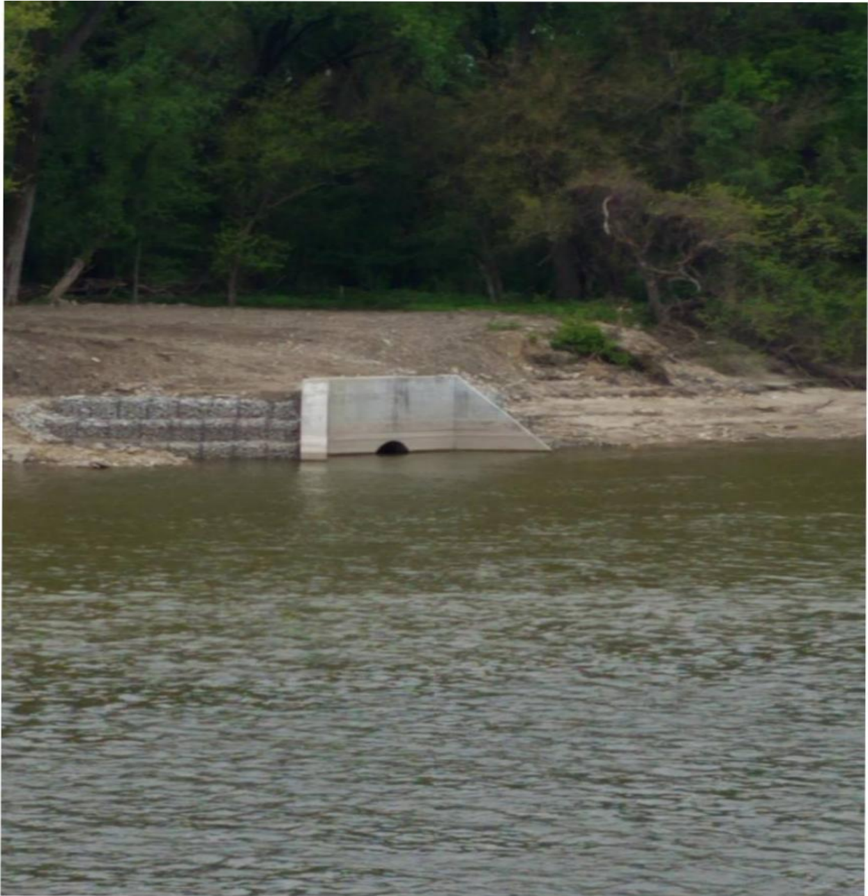
S.E. 4th and Van Buren Storm Water Pump Station Improvements
