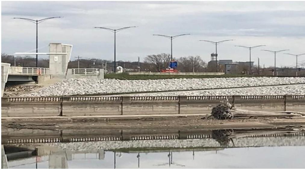
Southside MLK Bridge
