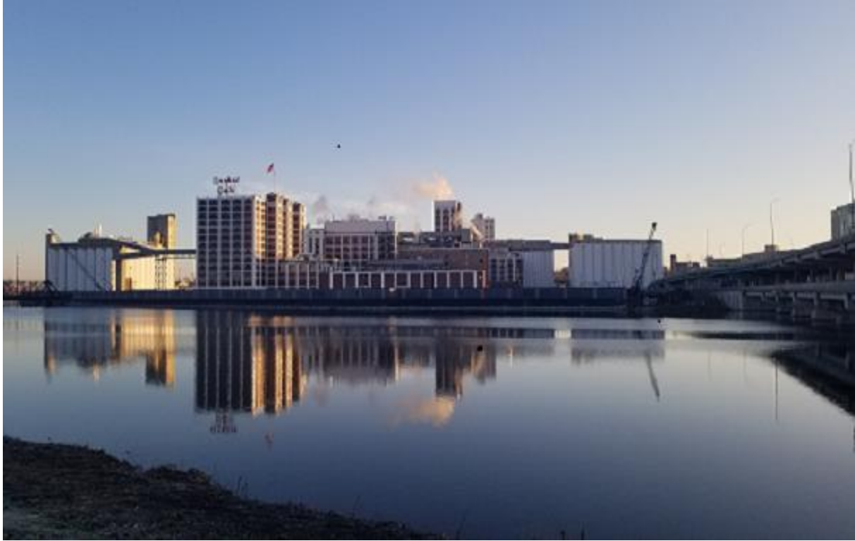
Quaker Oats Flood Wall – November 2020
