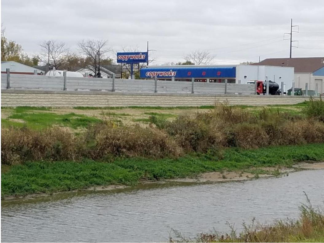
Figure 1: Floodwall west of Pump Station 10 as viewed from the north side of Clear Creek
