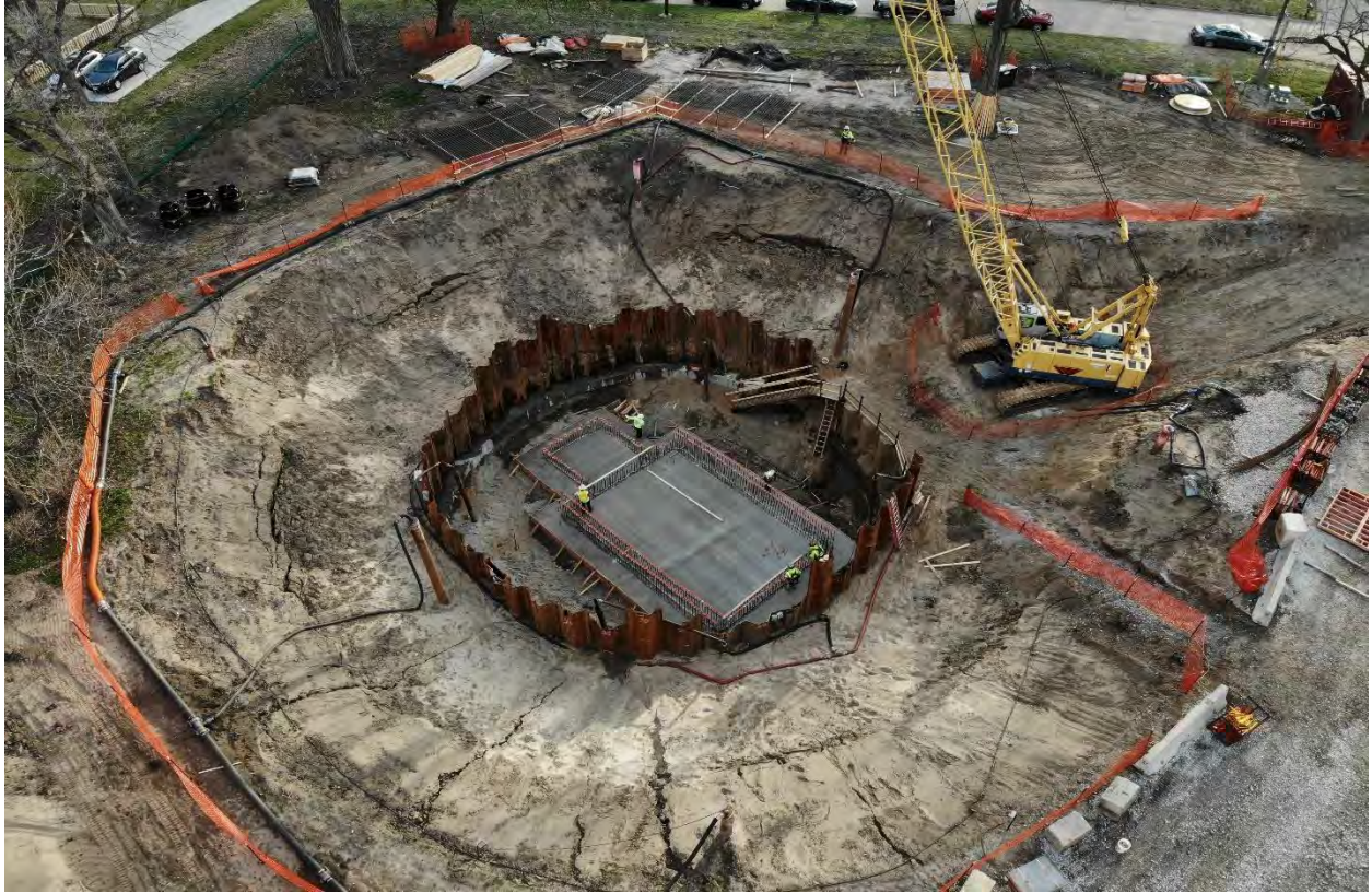
S.E. 9th Street Storm Water Pump Station and Improvements
