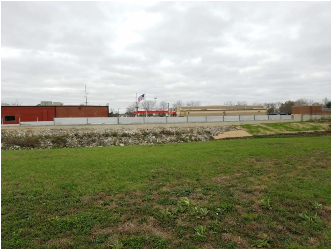
Figure 2: Floodwall east of Pump Station 10 as viewed from the north side of Clear Creek
